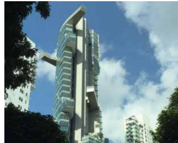
Project / RESIDENTIAL ARDMORE Place / SINGAPORE
