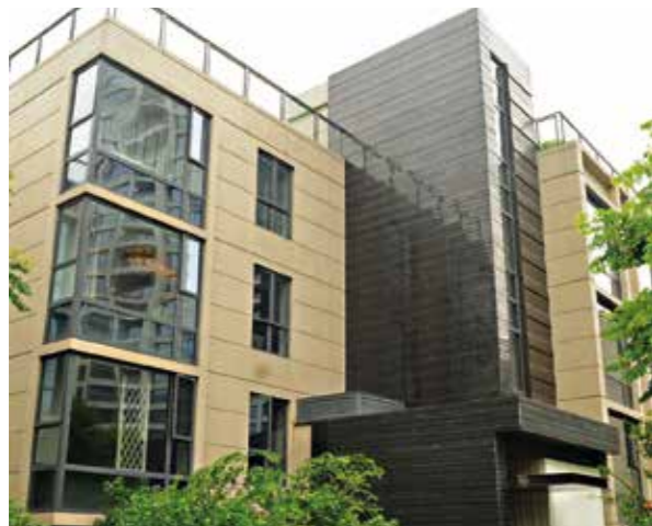
Project / RESIDENTIAL LAKEVILLE Place / SHANGHAI
